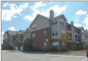
Archstone at River Edge 4825 Cameron Ridge Drive Indianapolis, IN
